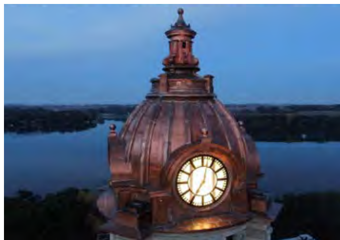
Martin County Courthouse
