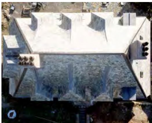
Yellowsands Thurlstone - Spojené kráľovstvo, Fa. Stuart Wheeler Roofing Ltd - Bodmin, Cornwall
